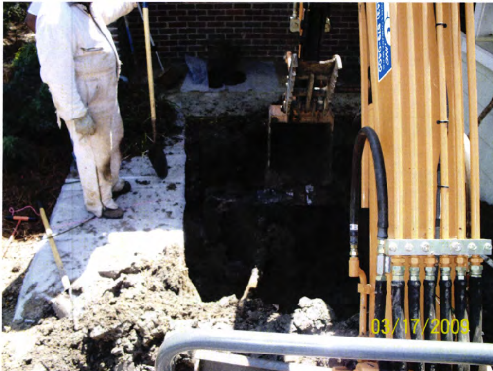
Picture 2: UST 140LaurelBayBlvd-1 being removed from the excavation.
