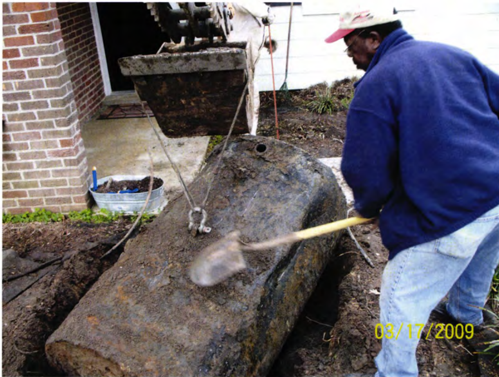
Picture 3: UST 140LaurelBayBlvd-2 being removed from the excavation.
